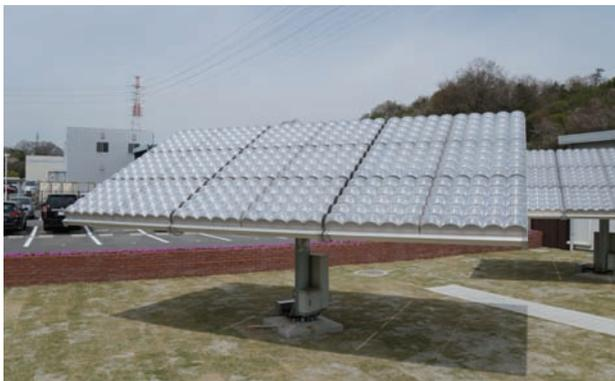
Fig. 14 Tracking-type solar power generation
