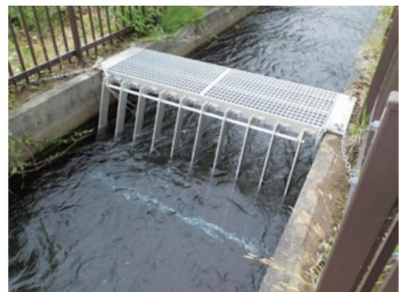
Fig. 12 Dust removal screen
