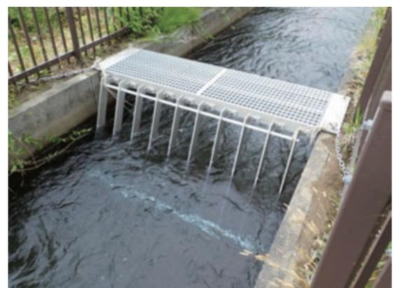
Fig. 12 Dust removal screen
