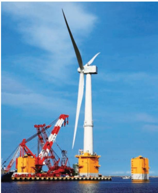
**Fig. 14** Largest-diameter wind turbine in world (diameter: 167 m, rated power: 7 MW, height of blade top: 189 m Courtesy : Toru Nagao)
