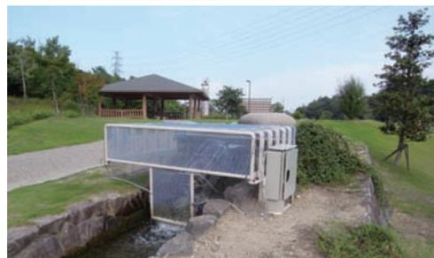
▲ Micro-hydropower generator installed in the nearby park (usually covered for safety as shown in the picture. p.6)
