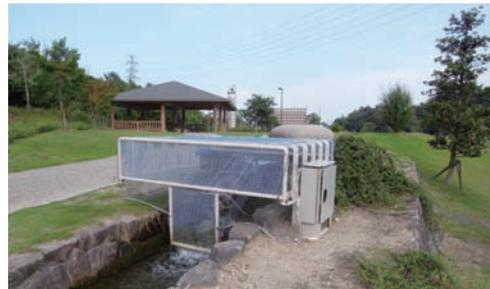
▲ Micro-hydropower generator installed in the nearby park (usually covered for safety as shown in the picture. p.6)
