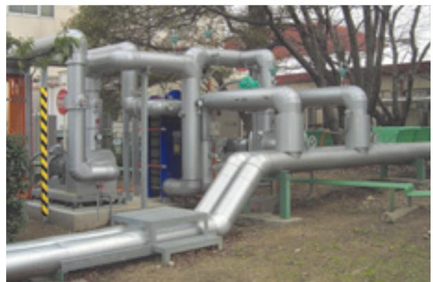
Fig. 4 Wastewater pipeline and heat exchanger at Iwata Works
