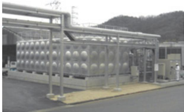
Fig. 6 A thermal storage tower for the new air conditioning system installed at Okayama Works
