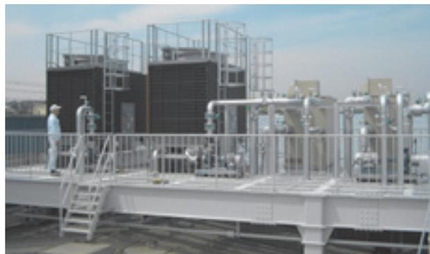
Fig. 7 Turbo refrigerator and cooling tower for the air-conditioning system at NTN Kongo Corporation
