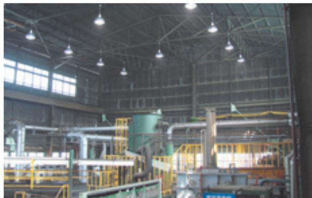
Fig. 8 Metal hydride lamps at a heat treatment plant of Kuwana Works
