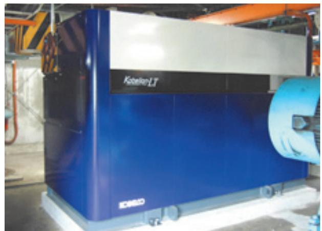
Fig. 5 High-efficiency screw compressor at Iwata Works
