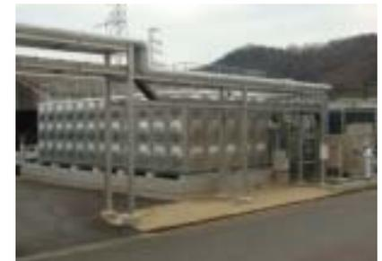
Thermal storage tank for hydrate-slurry air conditioning system (Okayama Works)
