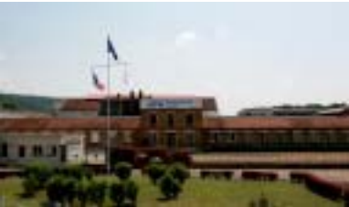
NTE Crézancy Plant (forging plant)
