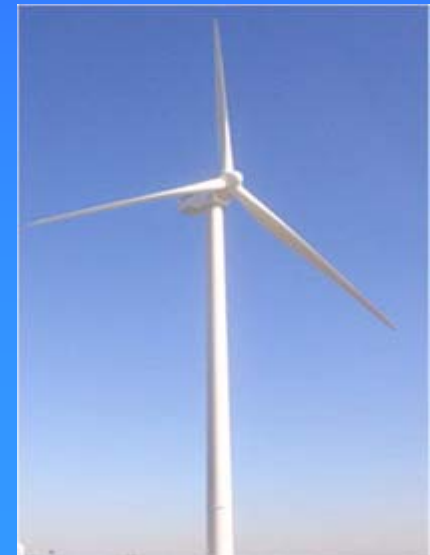
Large-size wind power generator
