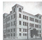
Old head office building
