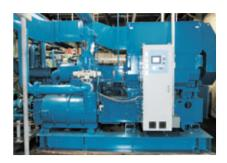
OKAYAMA Works is reducing its CO<sub>2</sub> emissions by upgrading to energy-efficient equipment. The company expects to reduce emissions by 1,560 tons annually through measures including installing high-efficiency air compressors and converting compressor cooling water pumps to inverter types.  $\Rightarrow p54$
