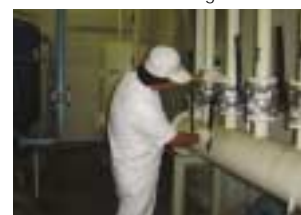
Checking for air leaks
