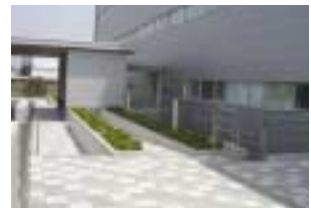
Walkway paving blocks made of waste media (grinding stones)
