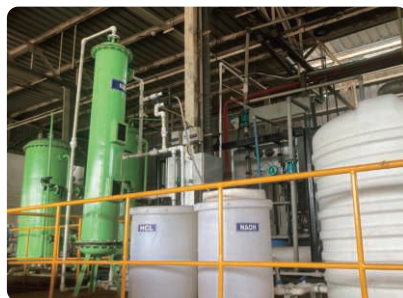
Dual-layer filtration water treatment facility tank and reverse osmosis (RO) water treatment facility (NNMI, India)
